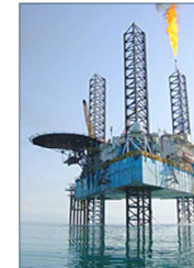
Figure 4: Soroosh Wellhead Platform 2 [Image courtesy of www.etech-group.co.uk]
