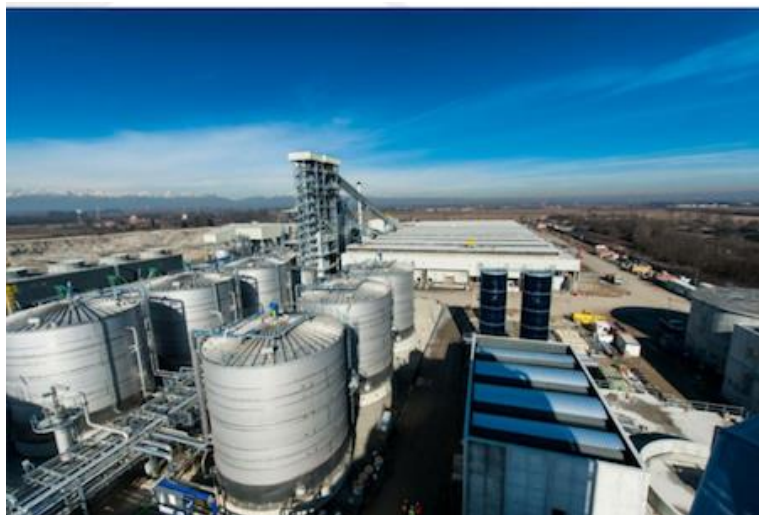
Figure 44: Chemtex facility (Crescentino, Italy, 20 mgy)
